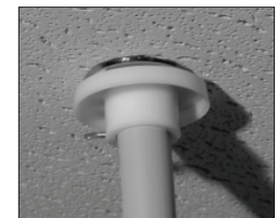
Figure 5: Correct use of the Cover Installer Tool
