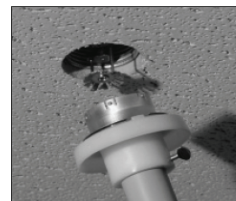
Figure 4: Use the Cover Installer Tool to install the Mirage® Concealed Cover Plate.
