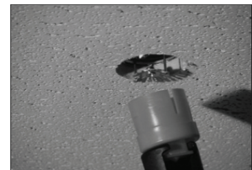
Figure 2: Use Sprinkler Wrench 14031 to remove the protective sprinkler cap.
